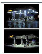
•Lighting should be in conformance with IESNA standards and utilize full cutoff luminaires.
